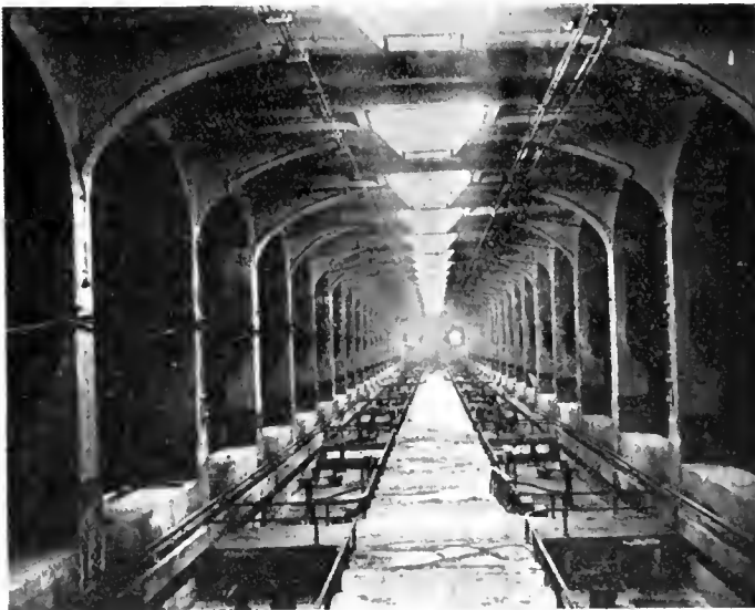
Fig. 8 - Final Filter Gallery.
